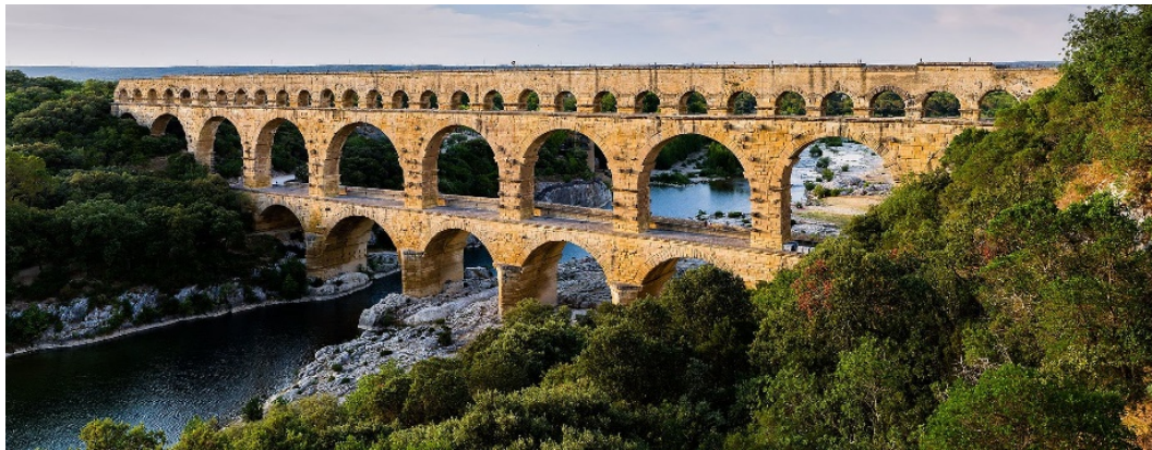
Figure 5.3. An example of Roman engineering skill, an ancient Roman aqueduct in South France build 2,000 years ago and functional for 900 years until maintenance was abandoned, but still standing.
